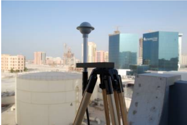
Figure 3: Installation outside at the Rayib Building showing the upper band probe
