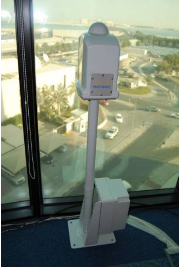
Figure 1: Installation of Insite Box at Taib Tower.
