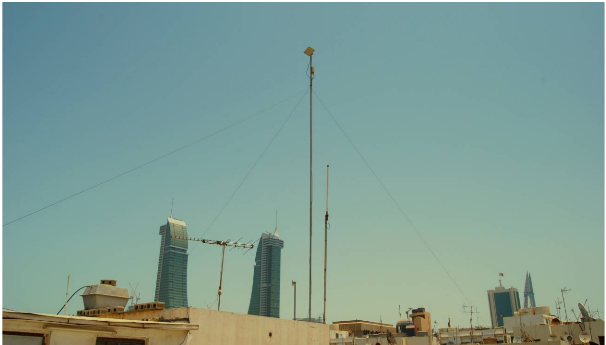
One of the illegal antennas
